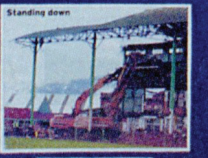
HIRIBIAN FOOTBALL CLUB Demolition of old stand 2000 (New stand opened 2001)
