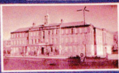
Front of Easter Road, Queen Margaret College (old Leith Academy buildings) taken in 1999. Photo: David Leverage
